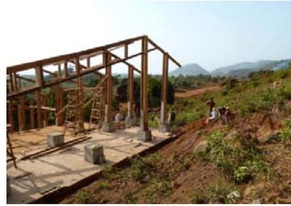
*16 March: BRELC with foundations, timber support columns and timber trusses.*
